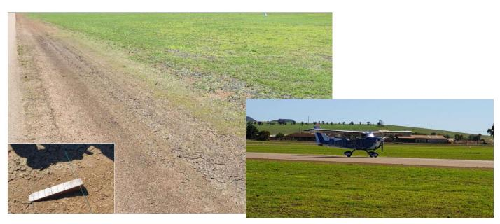
14/32 Runway Shoulder – surface cracking requiring resurfacing works
