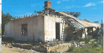
Above & to the left we see the extreme state of decay. The roof of 150 years ago had shingle cladding. But that was replaced a few decades later by corrugated iron when it became available. Inspection of the building shows nothing of historical value: The walls are standard poor stonework, and the roof is decayed typical jarrah framing, many, well preserved, examples of which exist today. So there is nothing remarkable, or in preservable condition
