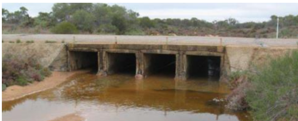
Photo 2: Culverts at Yuna Tenindewa Road over Hodgson Crossing)
