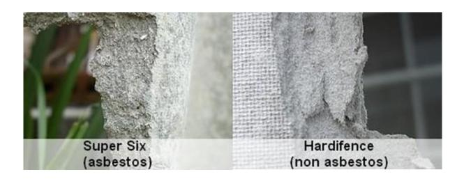
Warning: Do not break any suspect asbestos cement sheeting when taking a close up photo as this will release asbestos fibres which may be breathed in. It is safer to find an existing broken corner or edge to photograph.
