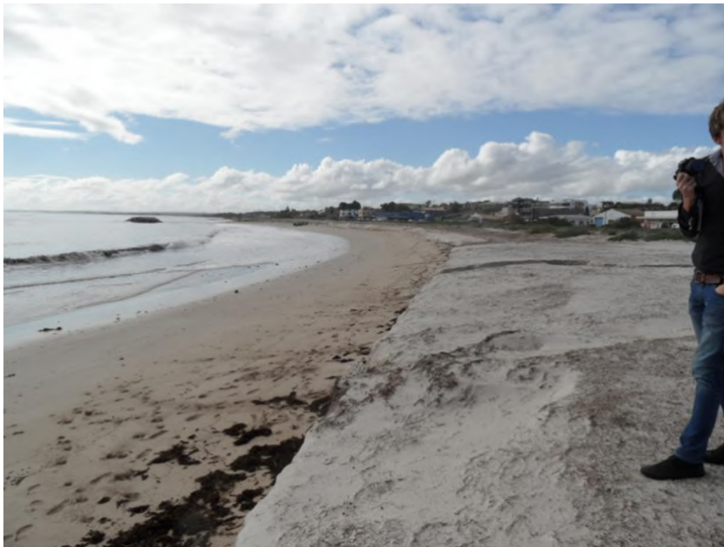
Figure 2.3: Erosion scarp at the southern end of the Beresford Foreshore - 30 June 2011
