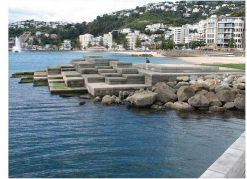
TYPE 2 HEADLAND - CONCRETE BLOCK EXAMPLE
