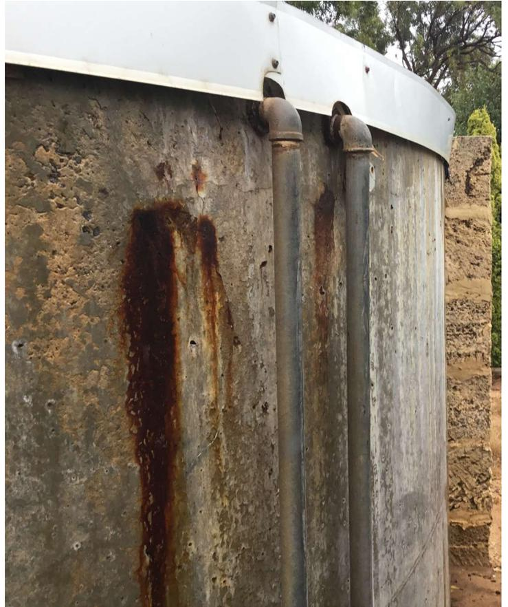
Apex Park Water Tank – severely corroded
