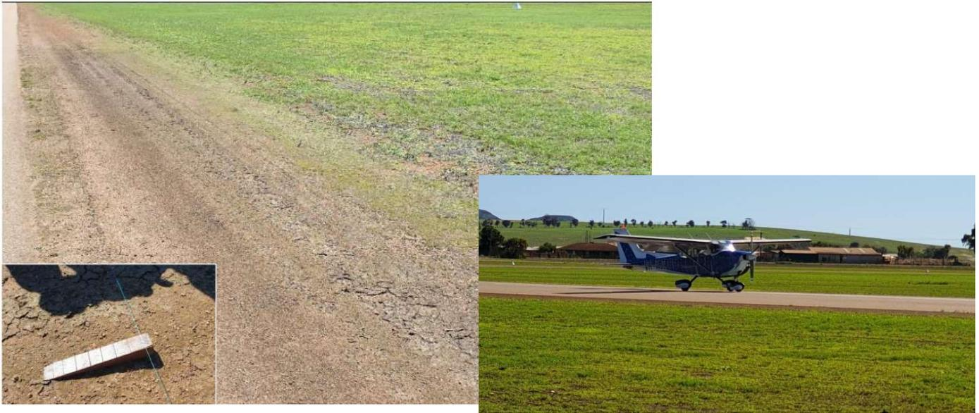
14/32 Runway Shoulder – surface cracking requiring resurfacing works
