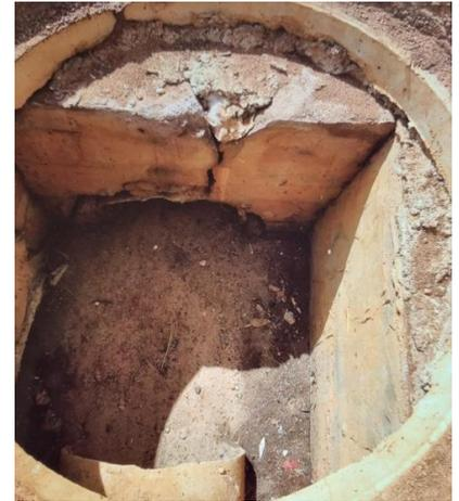
Drainage Renewals example (L-R): Corroded Manhole covers in the verge and cracked pit wall.
