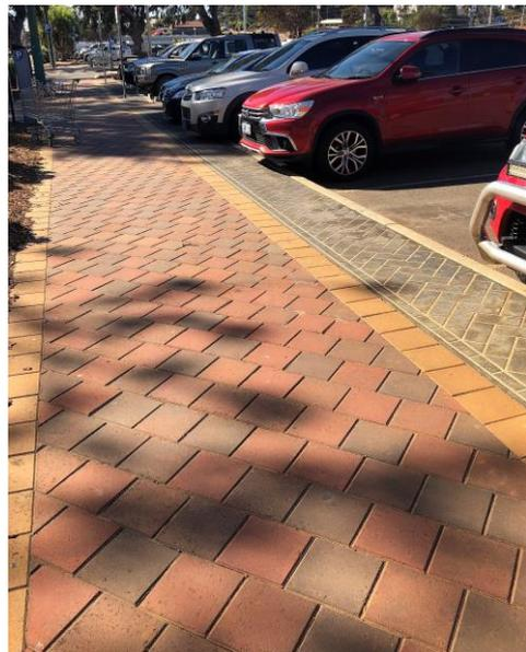
Wheel stops are often unnecessary and the 'overhang' area can be incorporated into an adjacent pedestrian path
