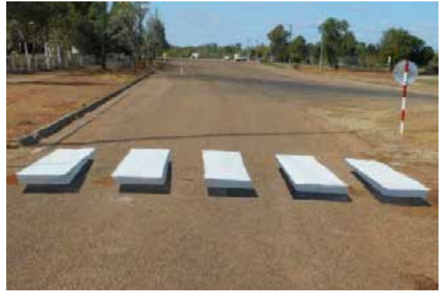
Figure 11 Examples of textural pedestrian crossing using line marking, signage, textures and speed cushion in Mt Hawthorn (top left); 3D painted zebra crossing in Boulia, Queensland (ABC News, 2018)(top right)
