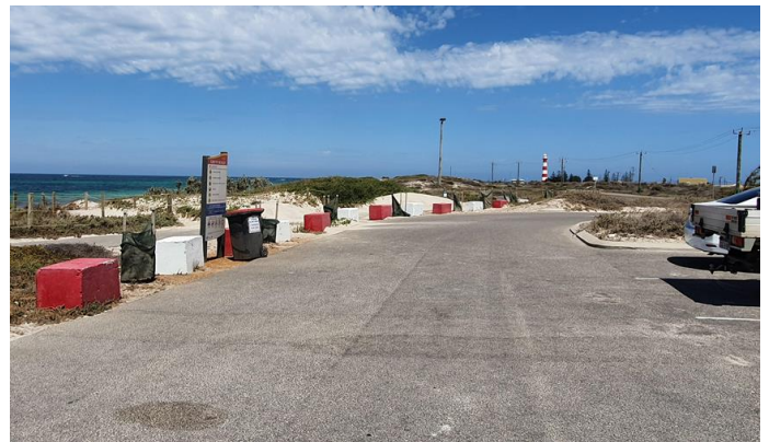
Parks & Gardens & Open Spaces – Greys Beach East Car park (renewal of bollards, fencing and landscaping in and around the carpark)
