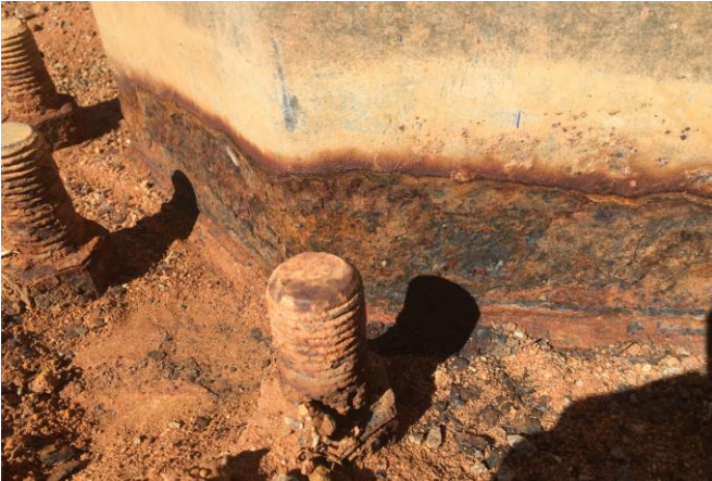
Example of corrosion at base of light poles
