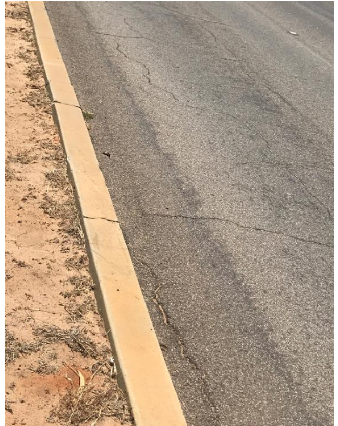
Renewal required Uta Karra Road (NWCH to Rifle Range Road)
