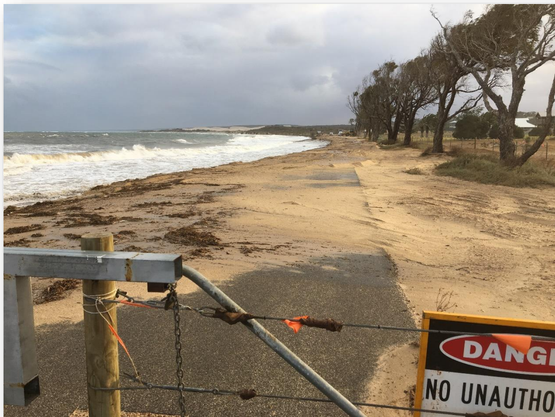
Image: The current condition of Whitehill Road.
