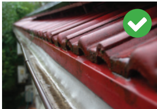
Well maintained gutter, clear of flammable material.
