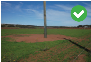
Power pole cleared 3m around base.
