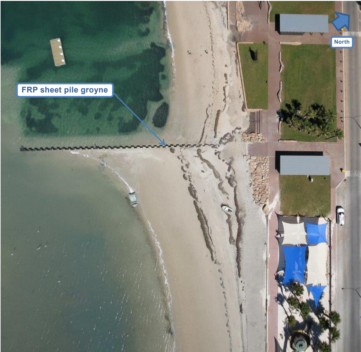
Figure 3.5 Denham Foreshore Composite Sheet Pile Groyne Aerial Photograph (Supplied by Department of Transport, 2016)
