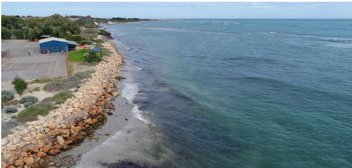
Figure 2.5 Ad-Hoc Seawall (Facing South)
