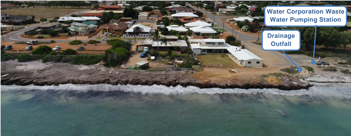
Figure 2.7 Infrastructure Adjacent to Coastline along Bluff Point North Site
