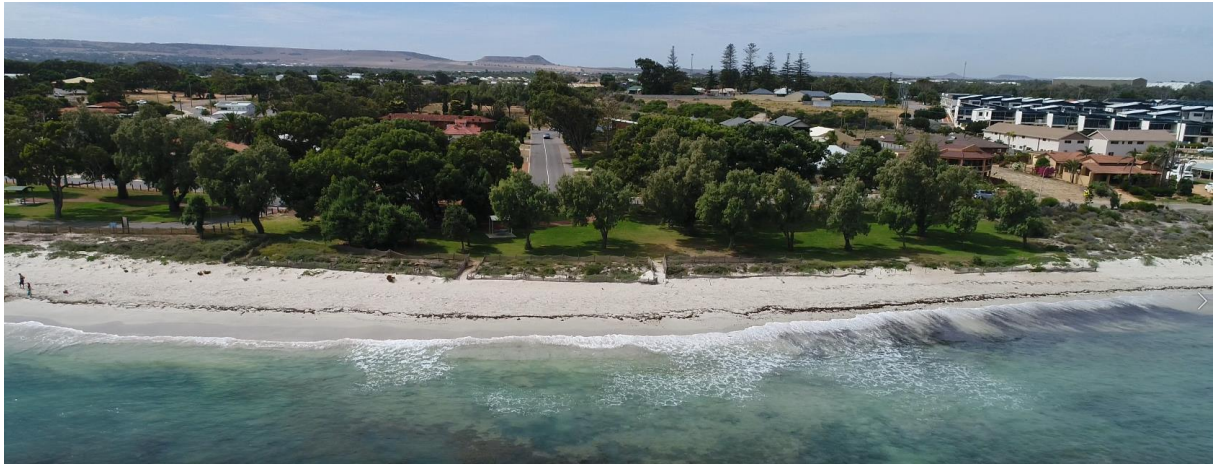
Figure 3.4 Wind Fencing at Bluff Point South
