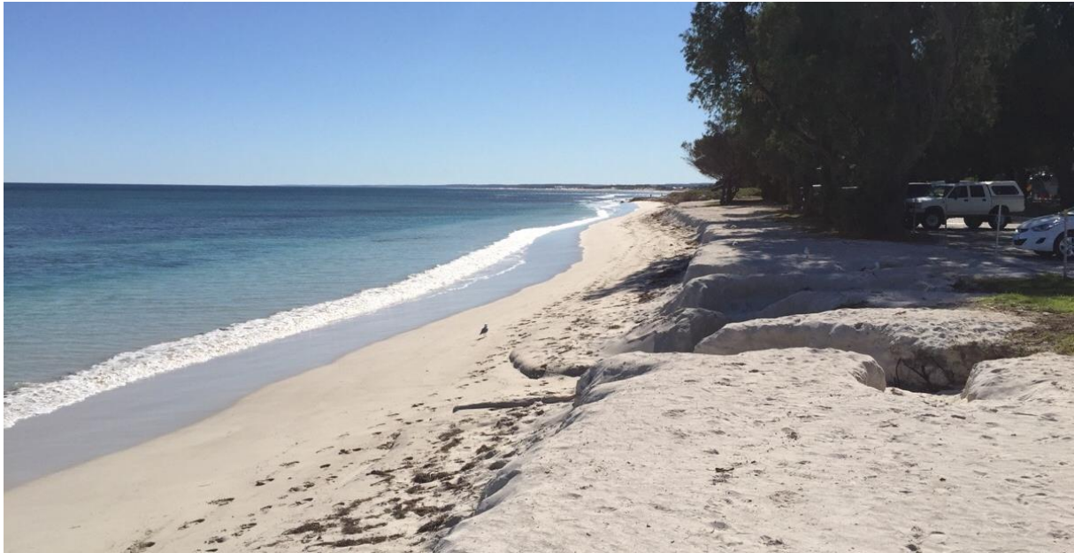
Figure 2.4 Photograph of Bluff Point South from July 2015 showing Eroded Profile
