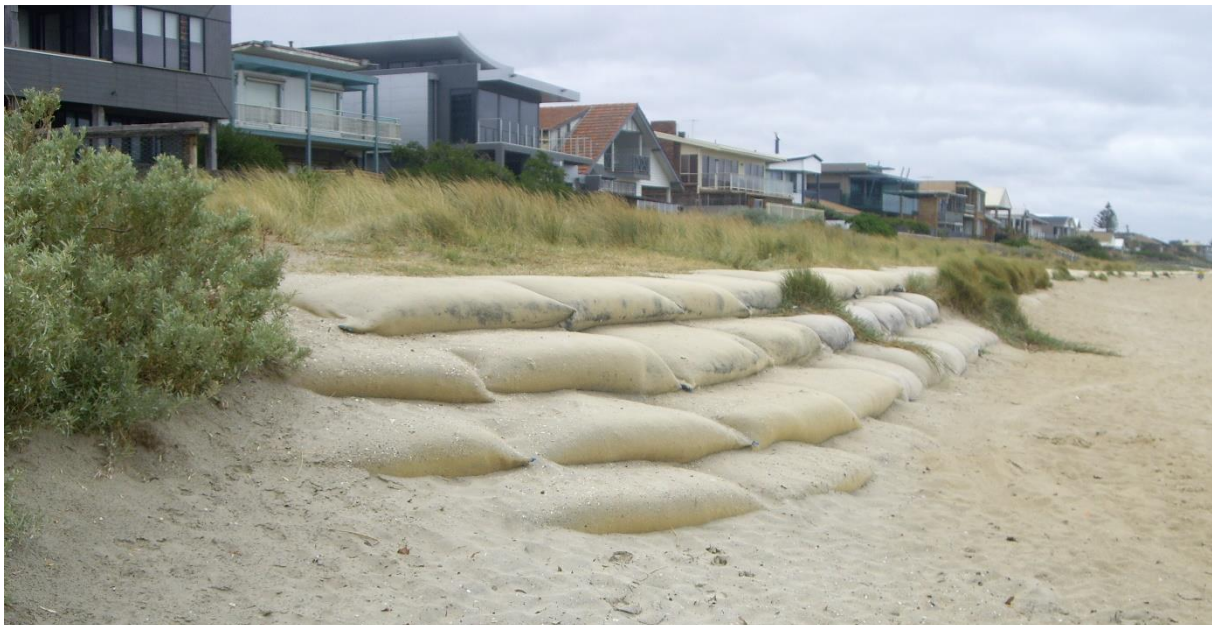
Figure 3.10 GSC Revetment Example
