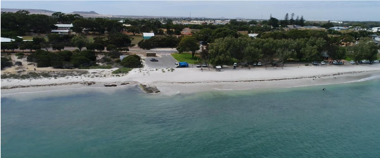
Figure 2.6 Oblique View of GSC Groyne
