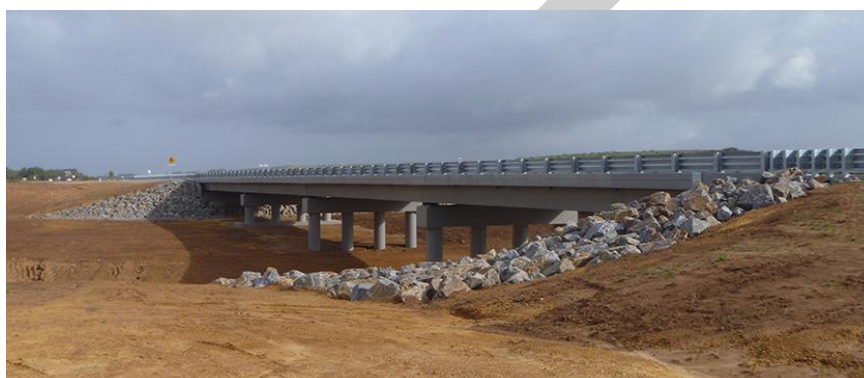
Figure 28 Greenough River Bridge replacement (Institution of Engineers Australia, 2014)
