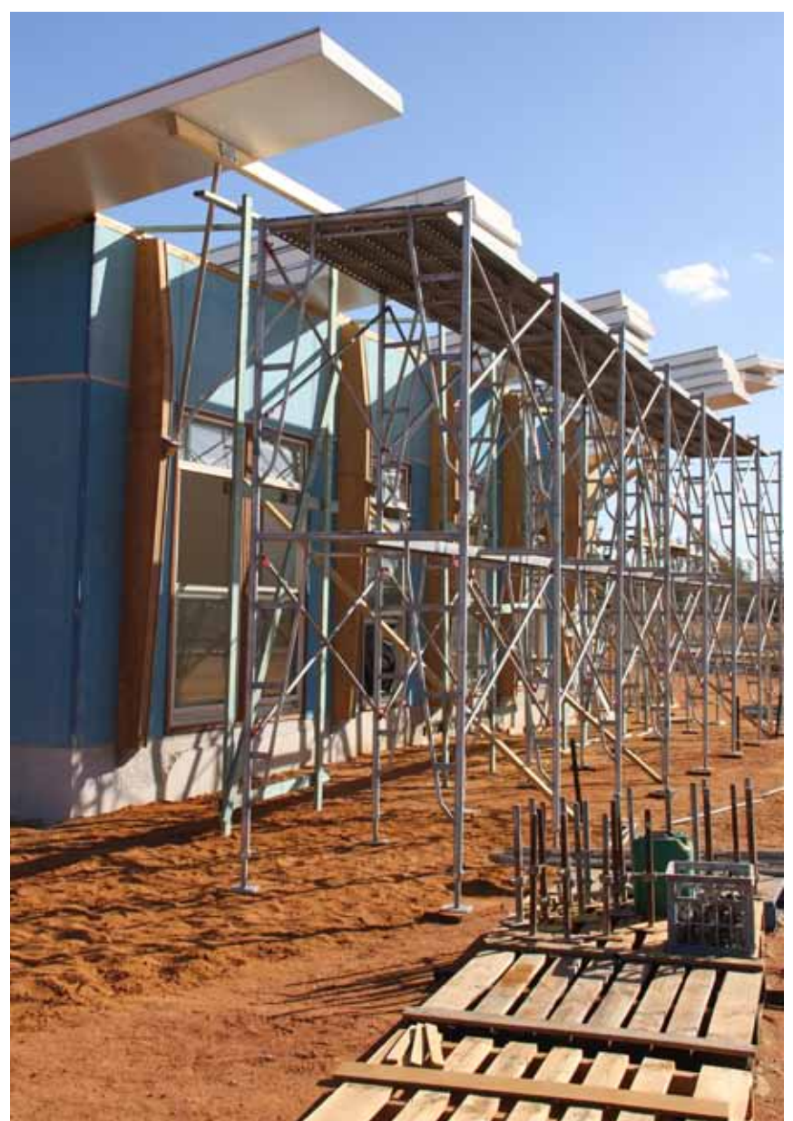
Perenjori flat pack housing pilot project
