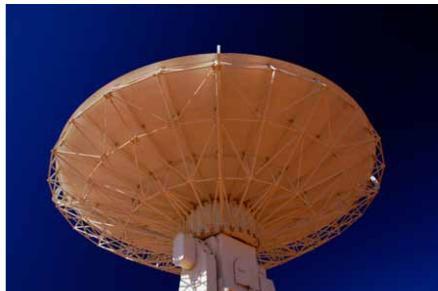
Square Kilometre Array antenna
