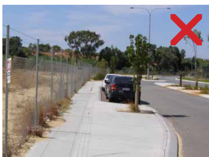
Example of a badly designed footpath within a car park. The path is narrow adjacent to the car bays and devoid of landscaping / shading.
