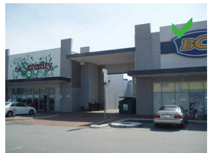
Service areas beyond the front facade.
