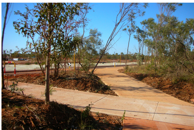
EXAMPLE OF VEGETATION BEING RETAINED IN ROAD RESERVE
