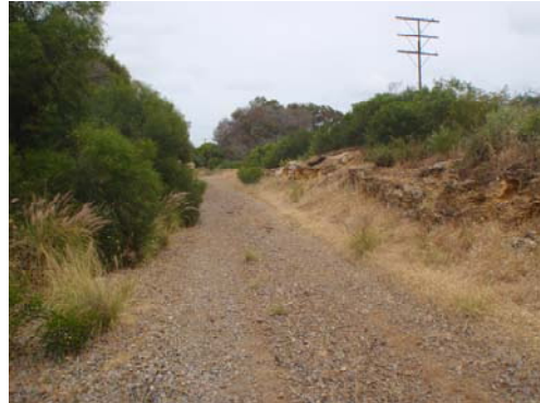
Swing Cut railway formation
