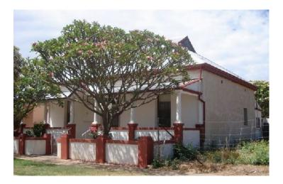
Photo Description: 11/12/2007 Rod Milne Verandah columns have replaced original posts.
