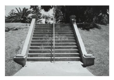
Photo Description: 8/12/1996 Suba & Grundy Low rendered masonry balustrade and central metal handrail.
