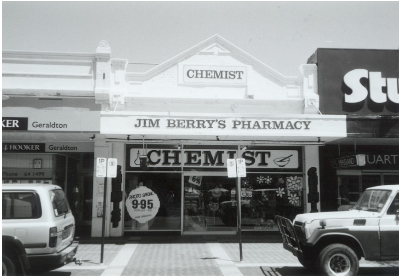
Photo Description: 8/12/1996 Suba & Grundy Modernised shop window.
