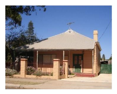
Photo Description: 31/10/2007 Rod Milne Cottage walls reclad with weatherboard.
