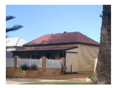
Photo Description: 3/12/2007 Rod Milne Corrugated iron wall cladding to side.
