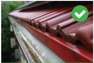
Well maintained gutter, clear of flammable material.
